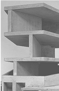
The Single - Wall Haus, Christian Kerez, Zurich, Switzerland, 2004 - 2007
