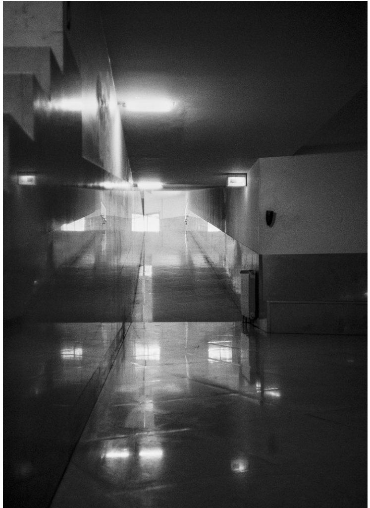
Fig. 13.1: Main ramp of the building B [Level 1]
