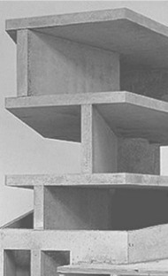
The Single - Wall Haus, Christian Kerez, Zürich, Switzerland, 2004 - 2007
